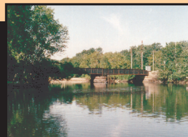
Railroad Trestle, Wolf River, New London
